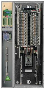
flown fixtures, LED lighting etc. This was a non-dim lighting panel, providing the needed circuits to support the complete lighting system.
